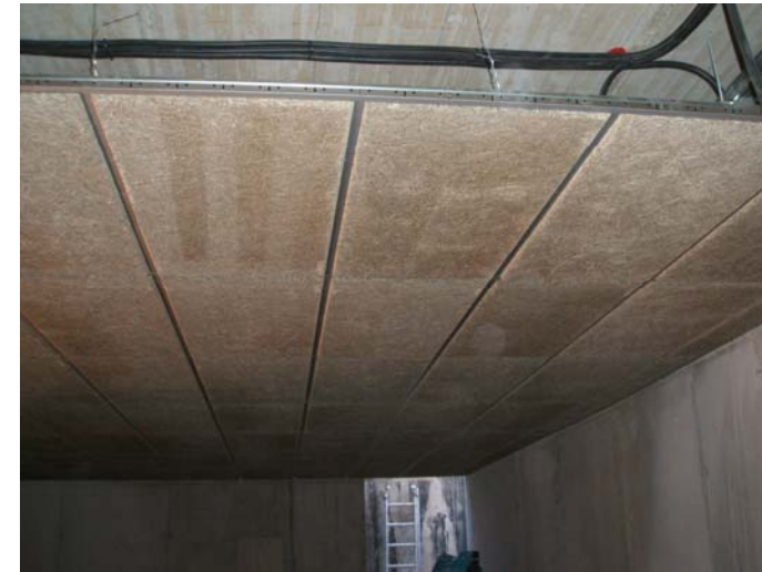
Fals sostre fonoabsorbent a la sala polivalent.
